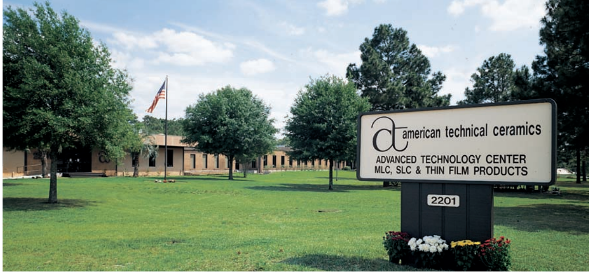
ATC Advanced Technology Center - Jacksonville, Florida
